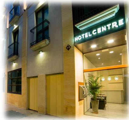
Hotel Centre Reus *** http://hotelcentrereus.com/home/
